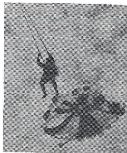
nected with sliding "D" rings on the front risers. Not being lashed down, they went too high on the risers and put the canopy below the jumper on several occasions. Photo by John Menzies.
